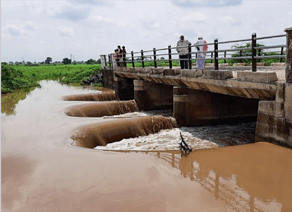
Bridge cum Bandhara, including Deck Slabs and Barriers between Piers
